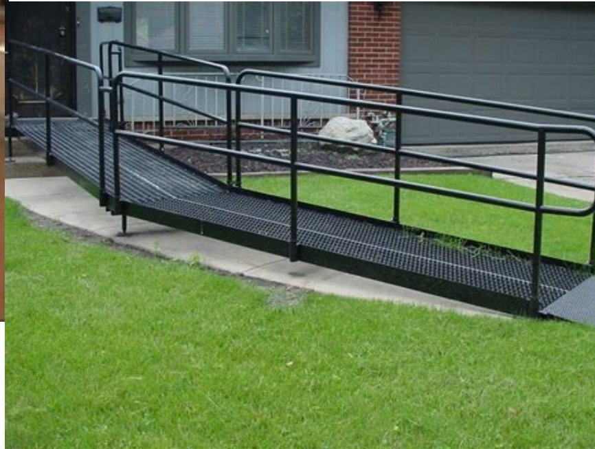
Input on equipment used with ramps
