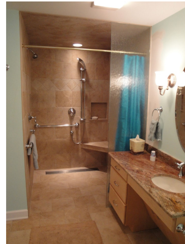
Placement of grab bars and sensor faucets
